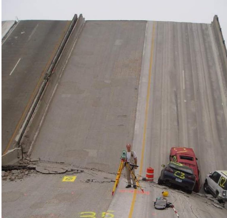
A forensic surveyor prepares to document a section of the I-35 Bridge Collapse in Minneapolis, Minnesota
