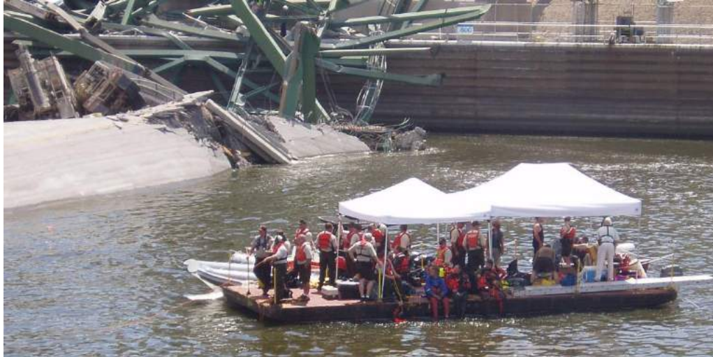
Dive operations in the Mississippi River at the collapsed I-35 Bridge in Minneapolis, Minnesota
